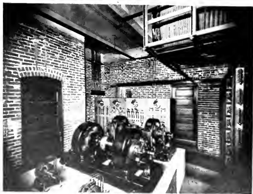
FIG. 10.—POWER PLANT, EAST BRANCH EXCHANGE.
